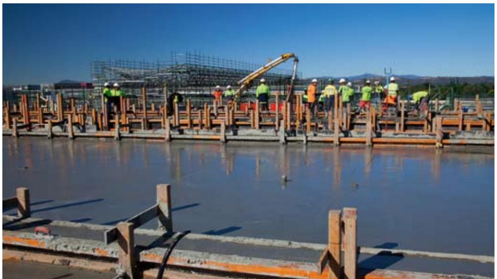
Top: The customary tree was erected at the highest point of the structure. Below: workers lay the final cement slab on the Southern Concourse Terminal.
