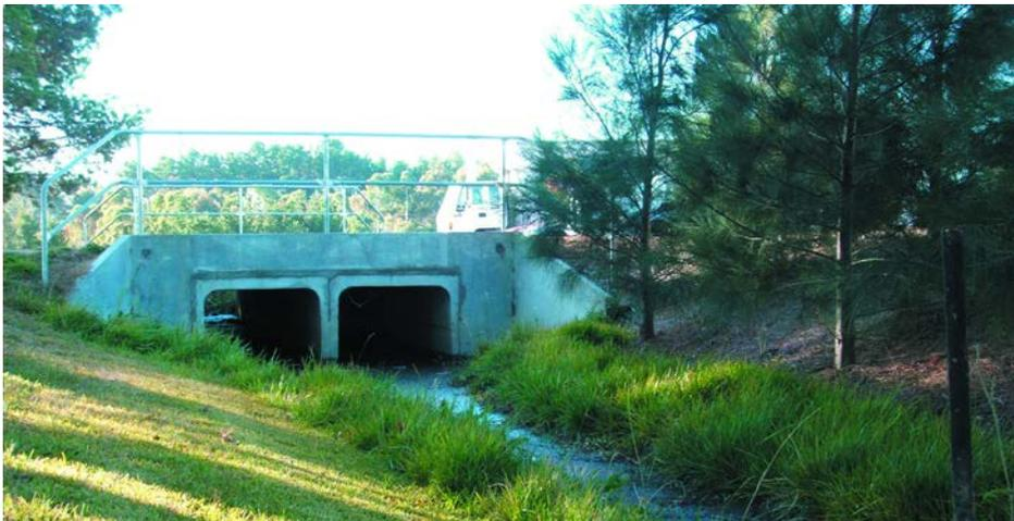
Photo 1: Concrete base designed to minimise turbidity in low fall swales
